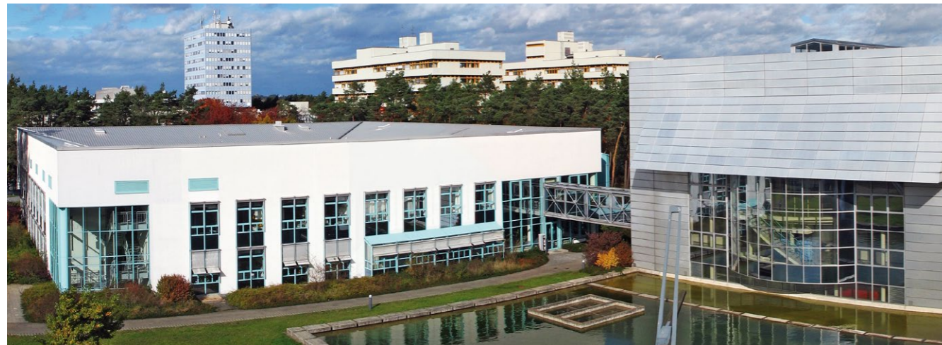
LEB building and cleanroom laboratory © Thomas Richter | Fraunhofer IISB
